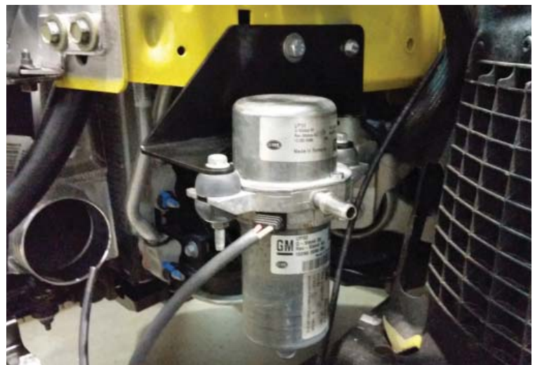
Brake Pump Relocated
