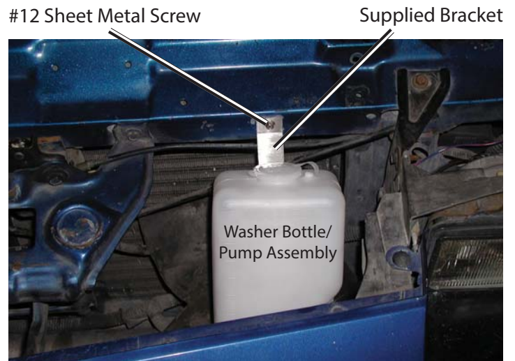
Supplied Washer Bottle/Pump Installed
