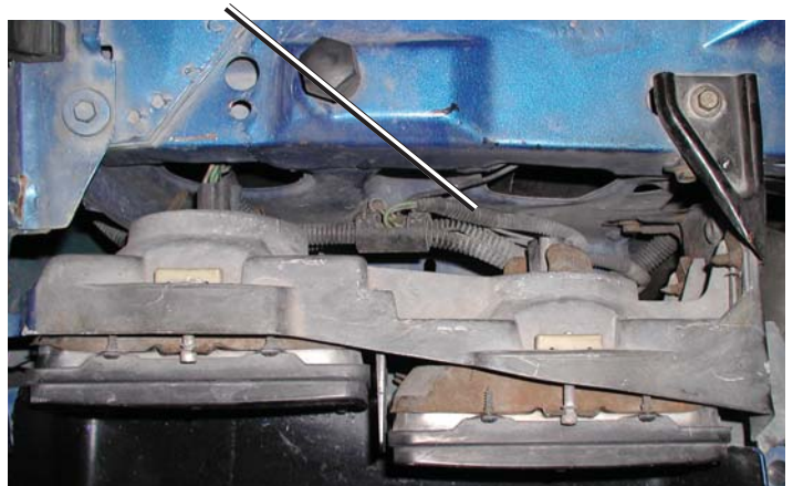
Wiring Harness Relocation (Pass. Side)
