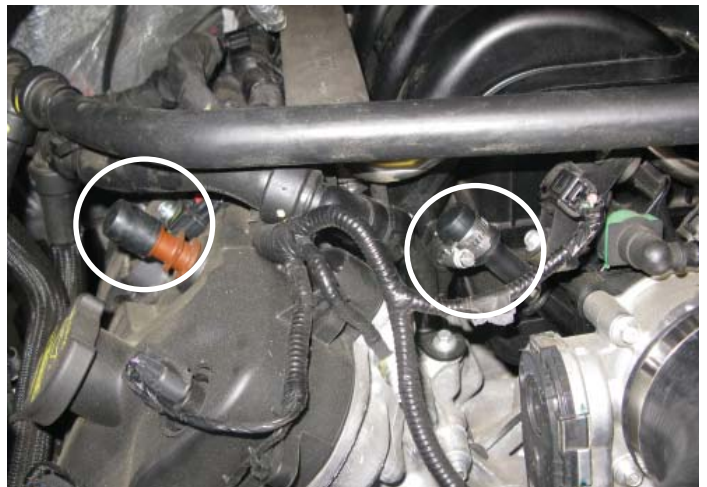
Rubber Caps Installed
