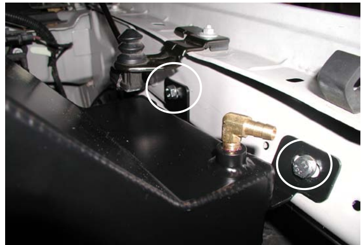
Coolant Tank Installed
