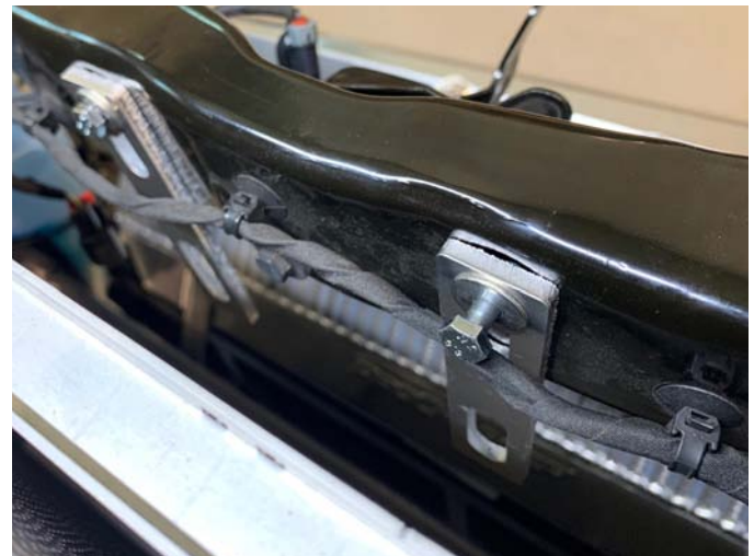
Upper Brackets Installed
