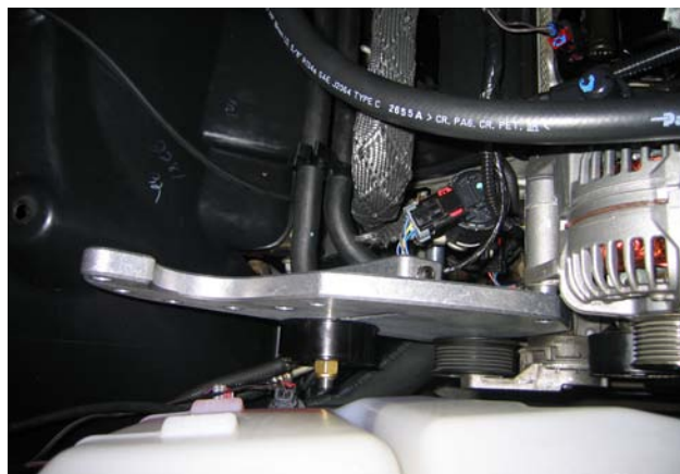
Main Bracket Installed
