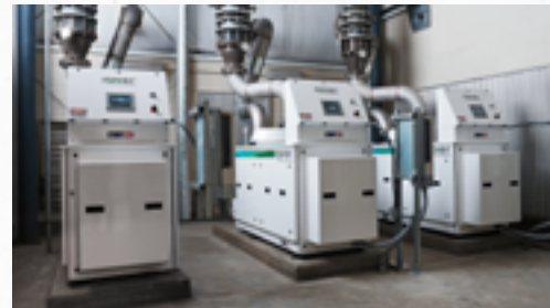
Inovair IM-20 Blower Packages at Midwestern Clean Water Plant
